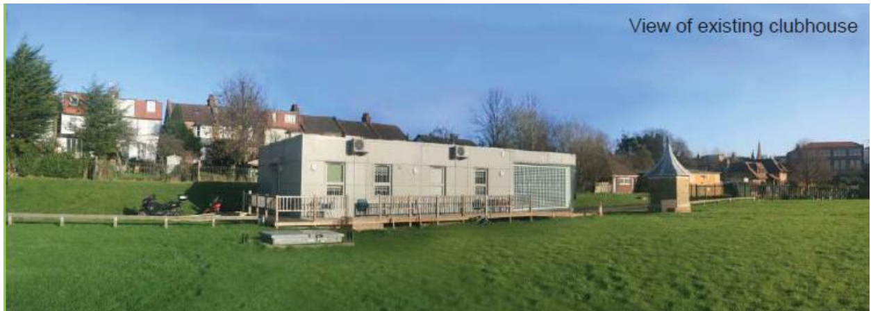
Current structure on site
